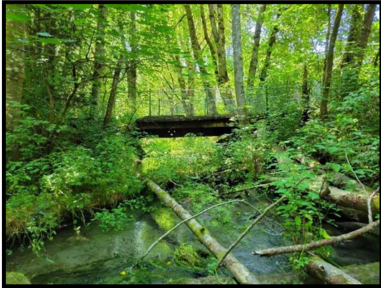
Figure 4: Pedestrian bridge approximately 490 feet upstream of the culvert inlet
