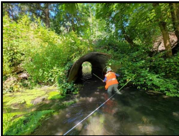
Figure 10: Culvert inlet at Draham St NE, facing downstream
