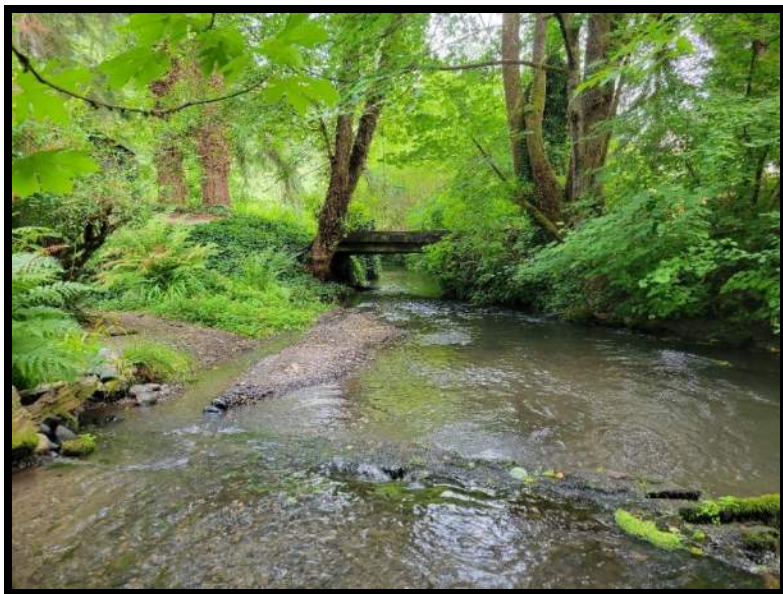
Figure 16: Existing private bridge approximately 400 feet downstream of the culvert outlet, looking downstream
