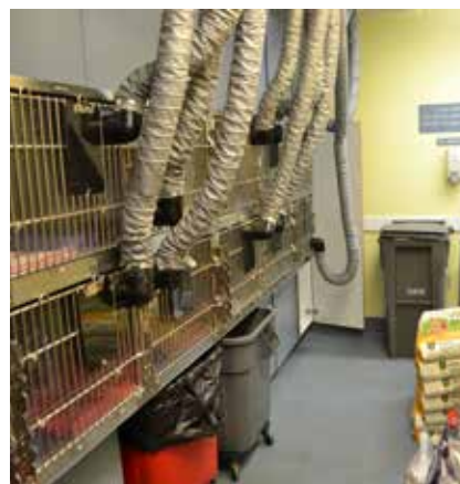
Figure 27. Ad hoc hoses are connected to kennels to provide adequate air circulation during isolation
