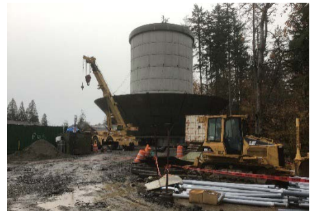
Constructing the Terry Cargil Reservoir
