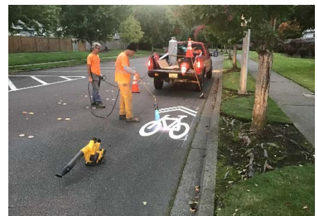
Applying shared lane thermoplastic bicycle symbols
