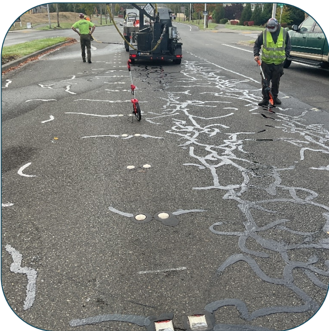
Fig. 16 Crack Seal @ Willamette Dr.
