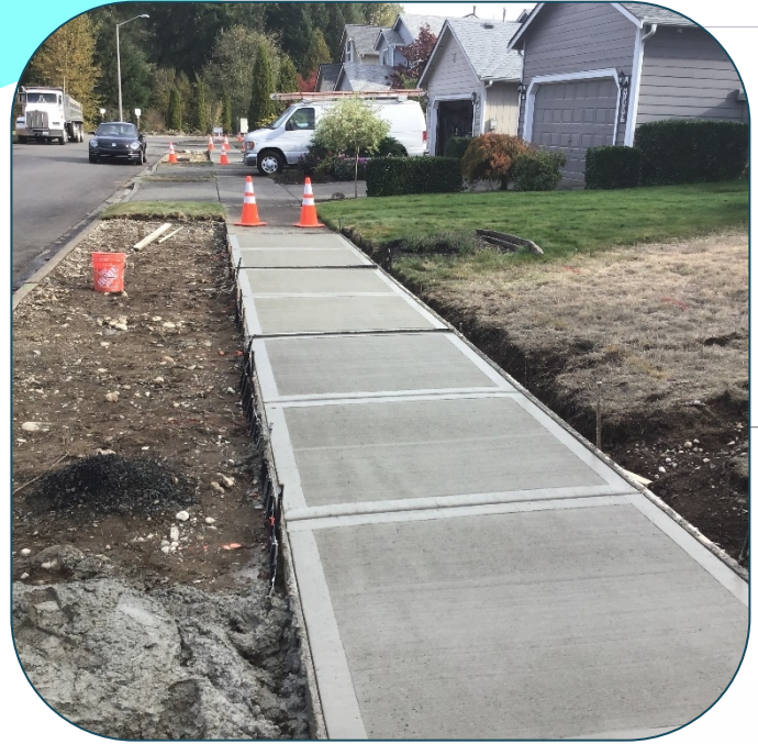
Fig. 15 Sidewalk @ Willows Crossing
