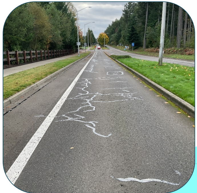
Fig. 17 Crack Seal @ 41 st Ave.
