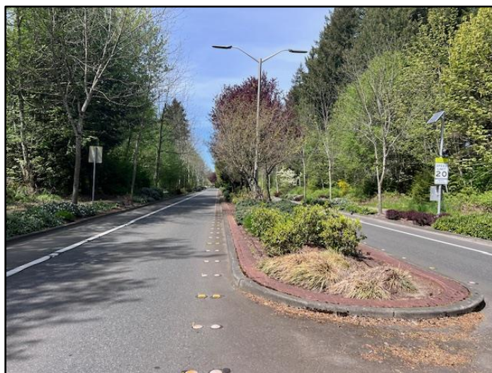
Mullen Rd, Looking NW
