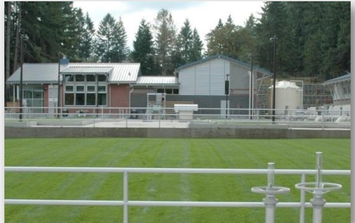
Martin Way Reclaimed Water Plant
