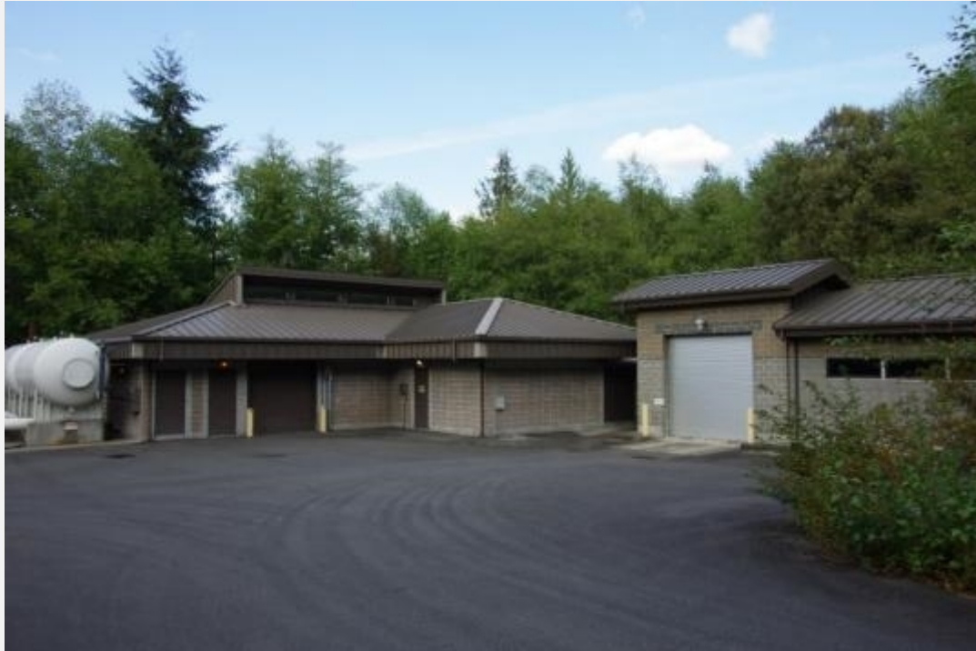
Martin Way Pump Station
