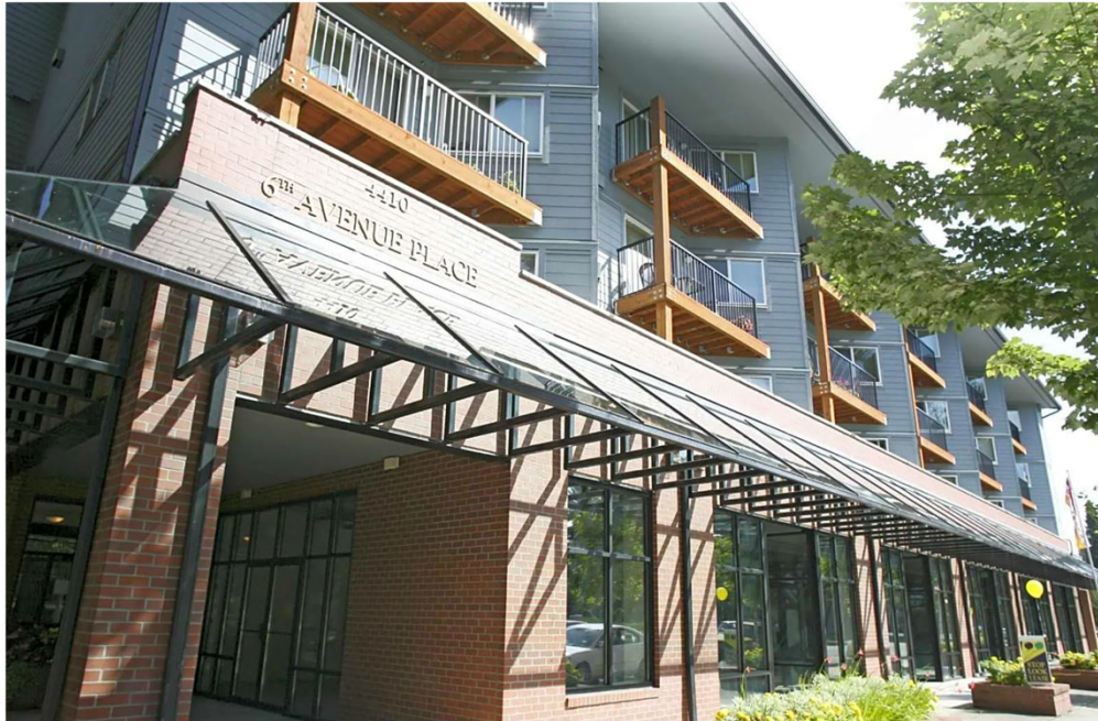
Live Work Units (initial build) 15 Feet GFH
