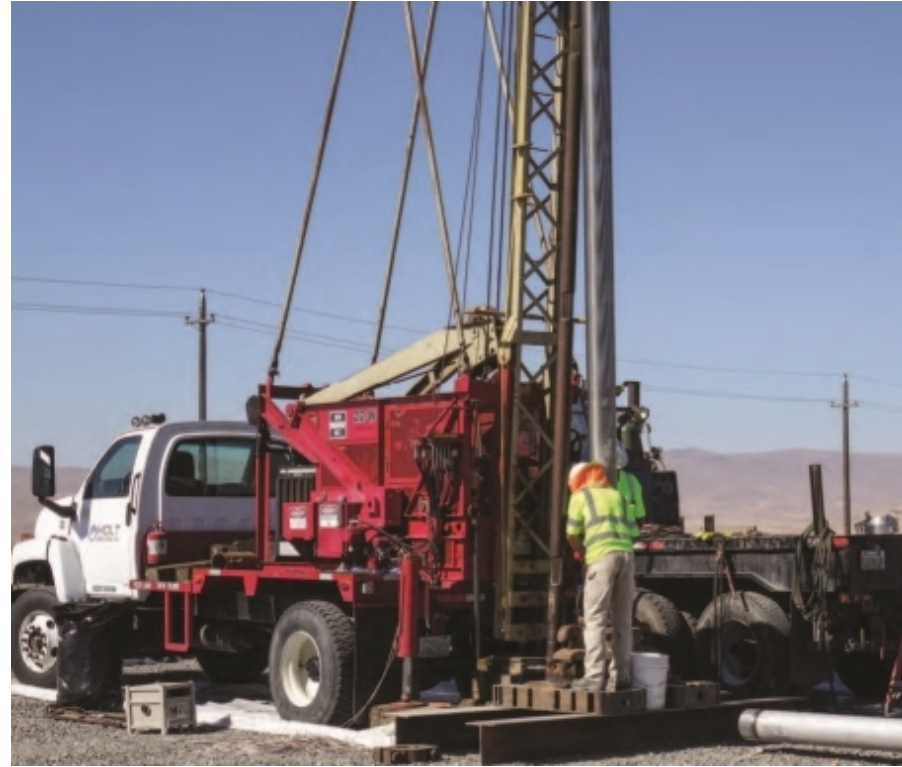
Typical Well Cable Tool Drilling Rig (460 to 750 ft deep)
