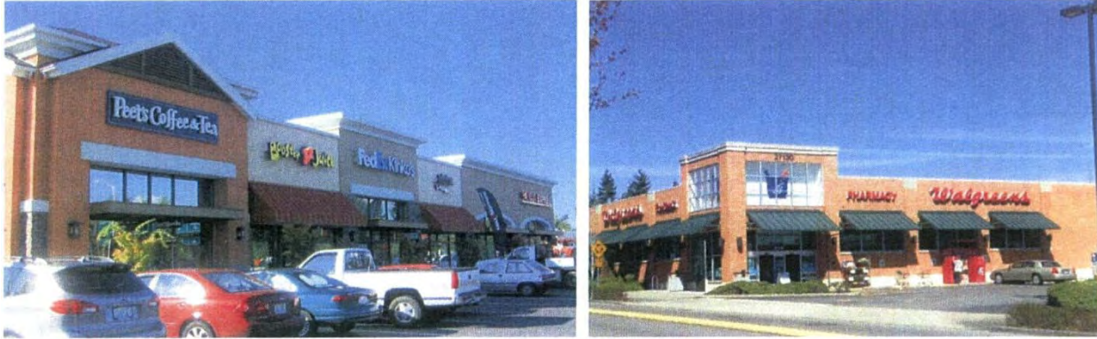
Figure 16.75.080(B)(3-2). More acceptable wall sign examples
