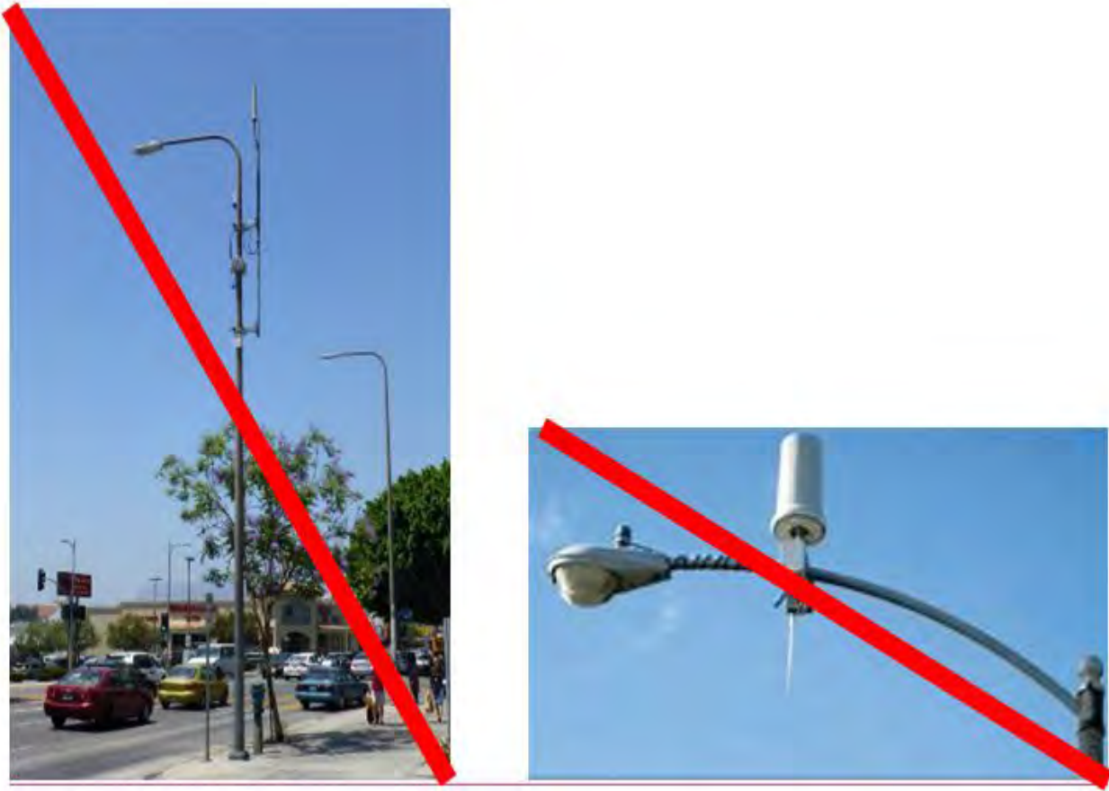
Figure 16.68.050(C)(4). Acceptable and unacceptable attachments
