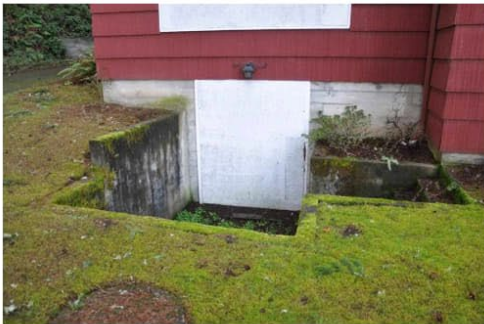
035 CloseUp of basement access.jpg
