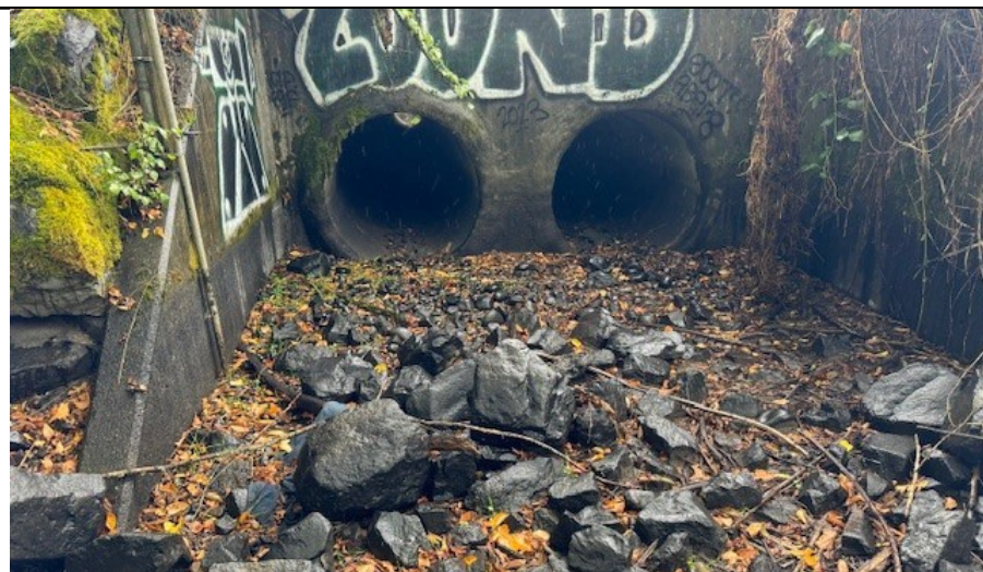
Photo 6. Facing southeast from the channel of Woodland Creek in the southernmost portion of the study area. The culverts are four feet in diameter and they span Pacific Avenue SE. October 2024.
