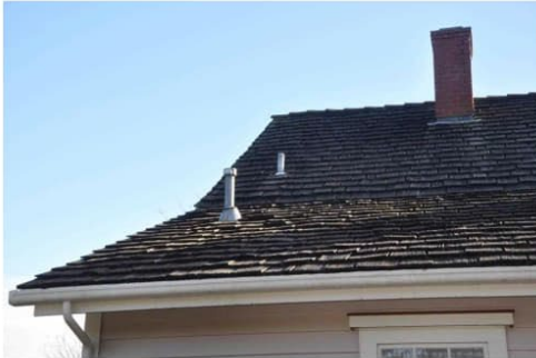
021 Roof of house.jpg
