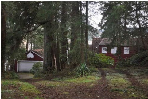
005 Driveway approach from SW.jpg
