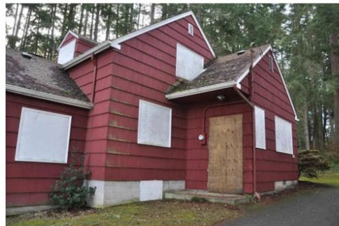
050 NE Entrance to house.jpg
