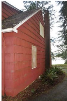
045 South side of house.jpg
