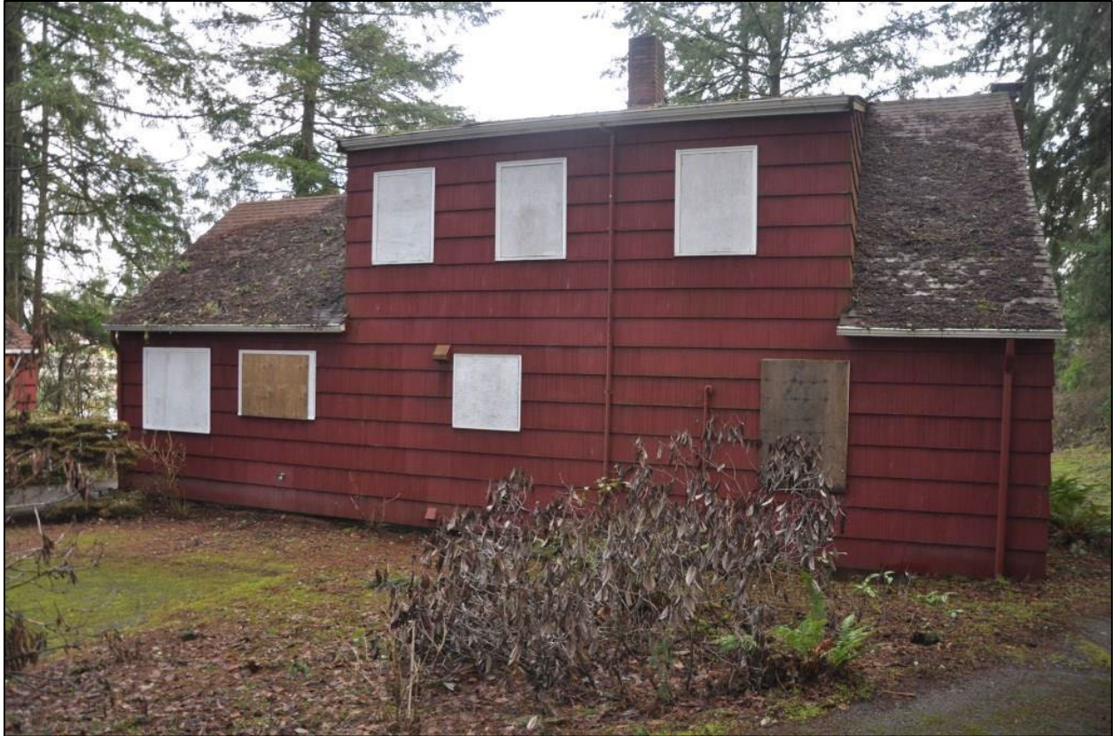
Photo 14. View of rear (west) façade, taken in 2025.
