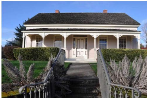
005 Front Facade facing NW.jpg
