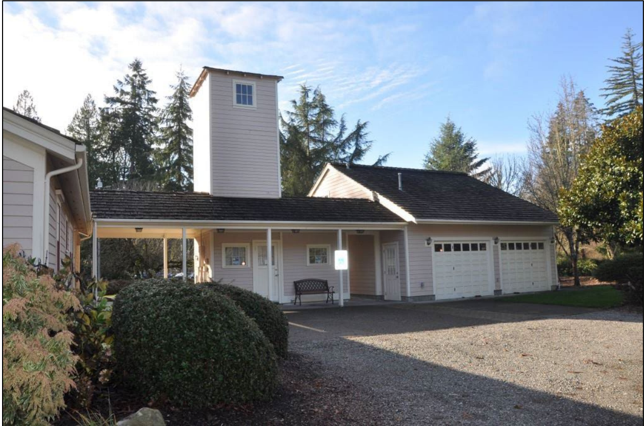
Photo 8. Water tower and detached garage apartment with breezeway, taken in 2025.
