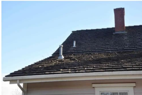
021 Roof of house.jpg
