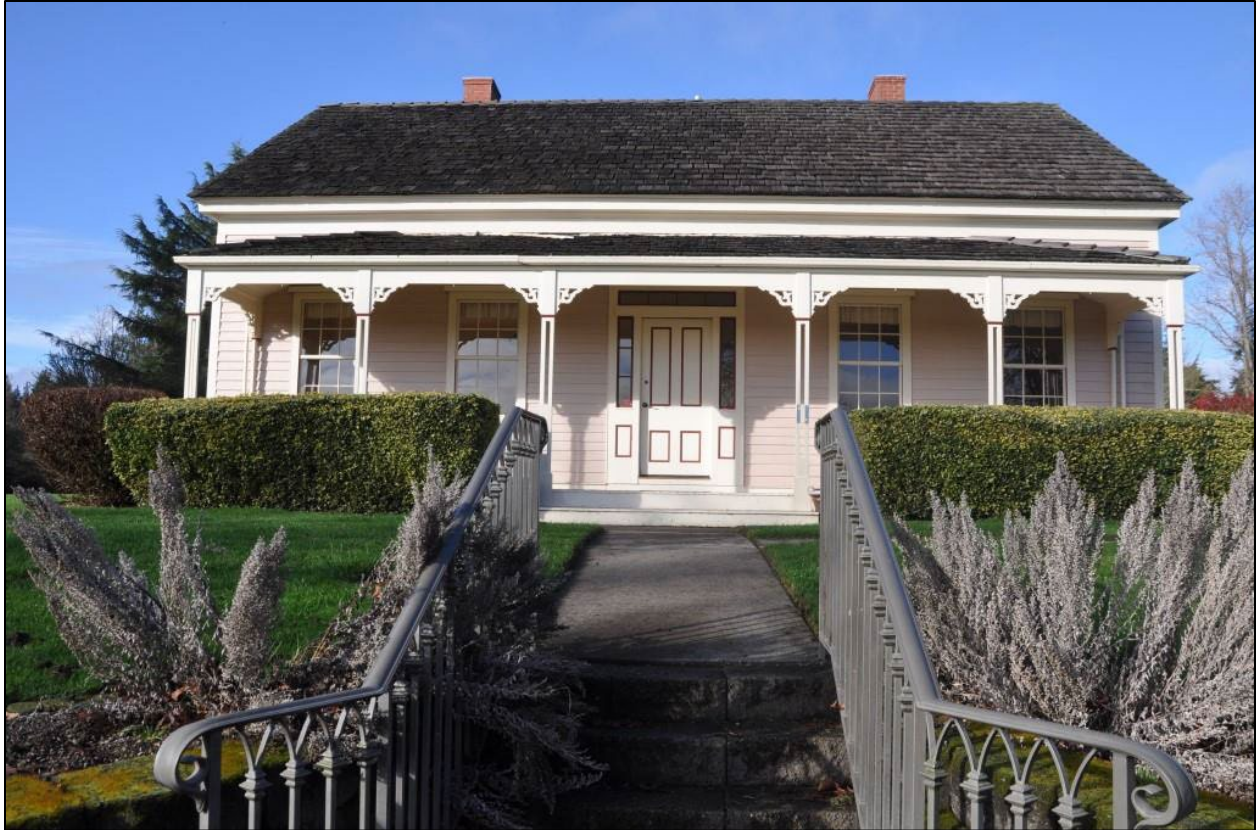
Photo 5. View of main façade (south), taken in February 2025.
