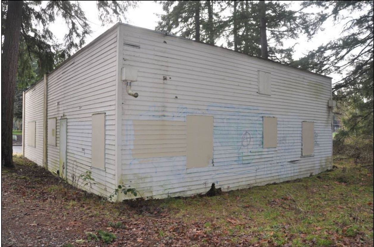
Photo 20. View of rear (north) façade and east façade. Taken in 2025.
