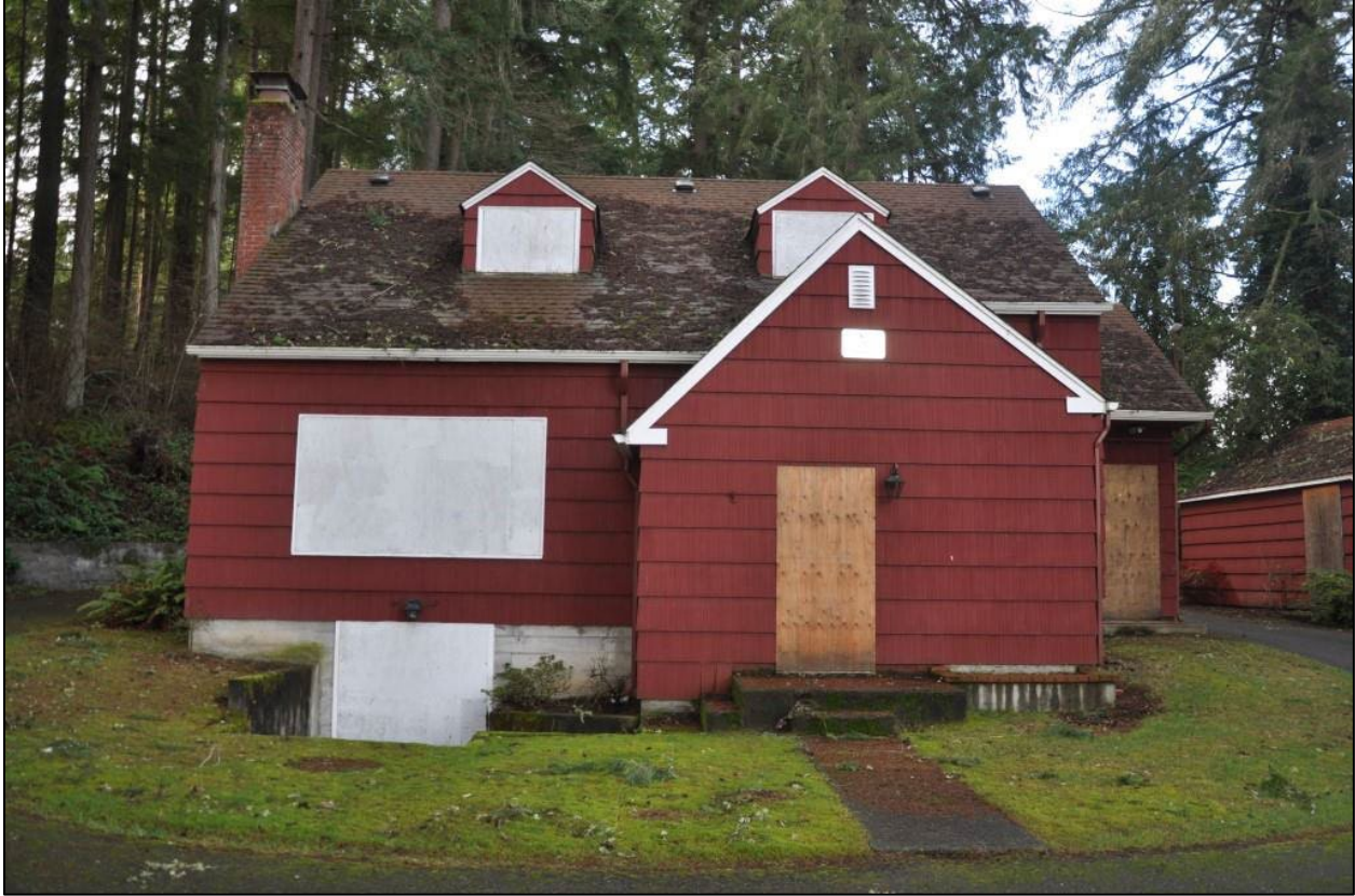
Photo 12. View of main (east) façade, note infill of windows and doors. Taken in 2025.
