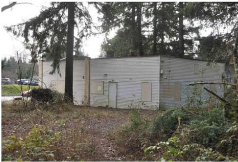
McKinney Building3 northeast corner showing side detail.jpg
