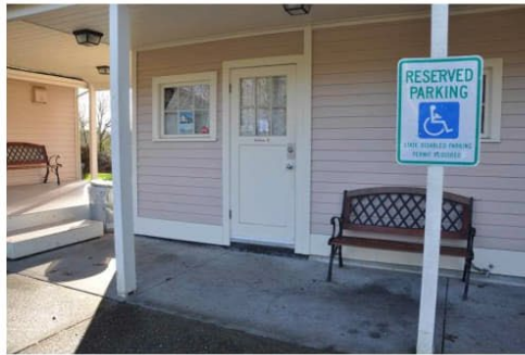
055 Tower Office Entrance facing SW.jpg
