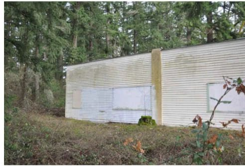
McKinney Building4 west side facing northeast.jpg
