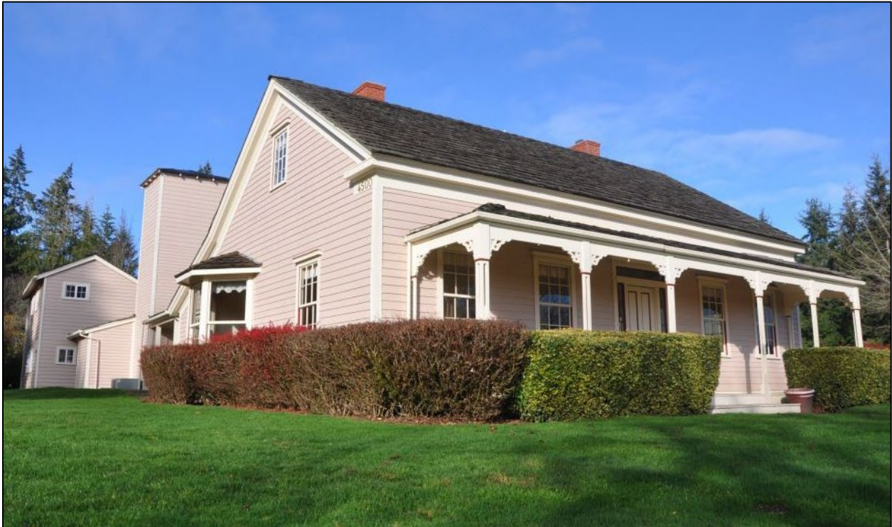
Photo 7. View of west façade with main façade and porch, taken in February 2025.
