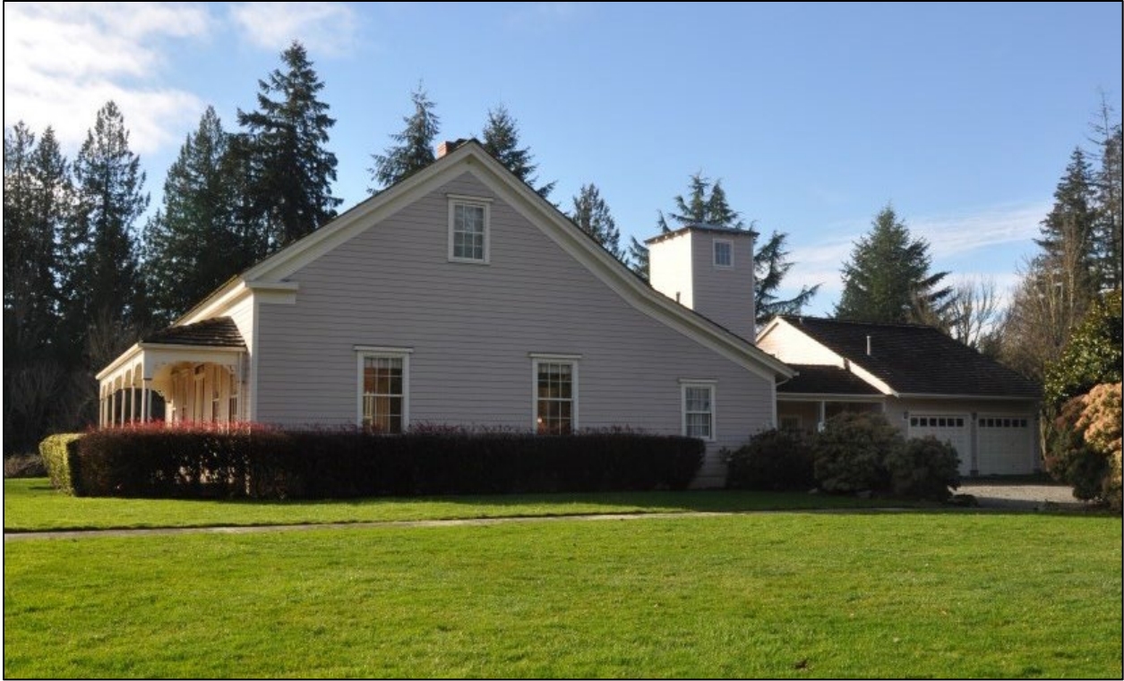
Photo 6. View of the east façade with water tower and detached garage. Taken February 2025.
