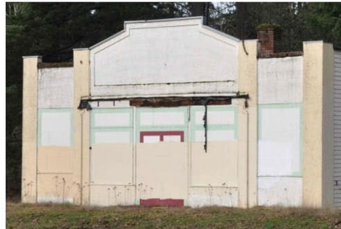
McKinney Building1.1 front facade closeup, view facing north.jpg
