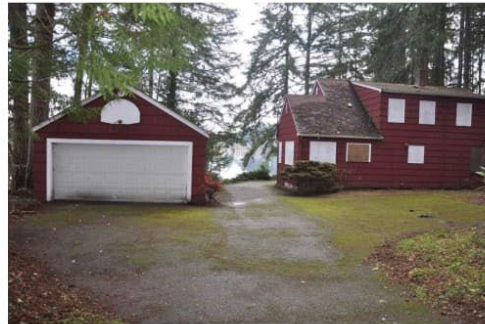
040 West side of garage with house.jpg
