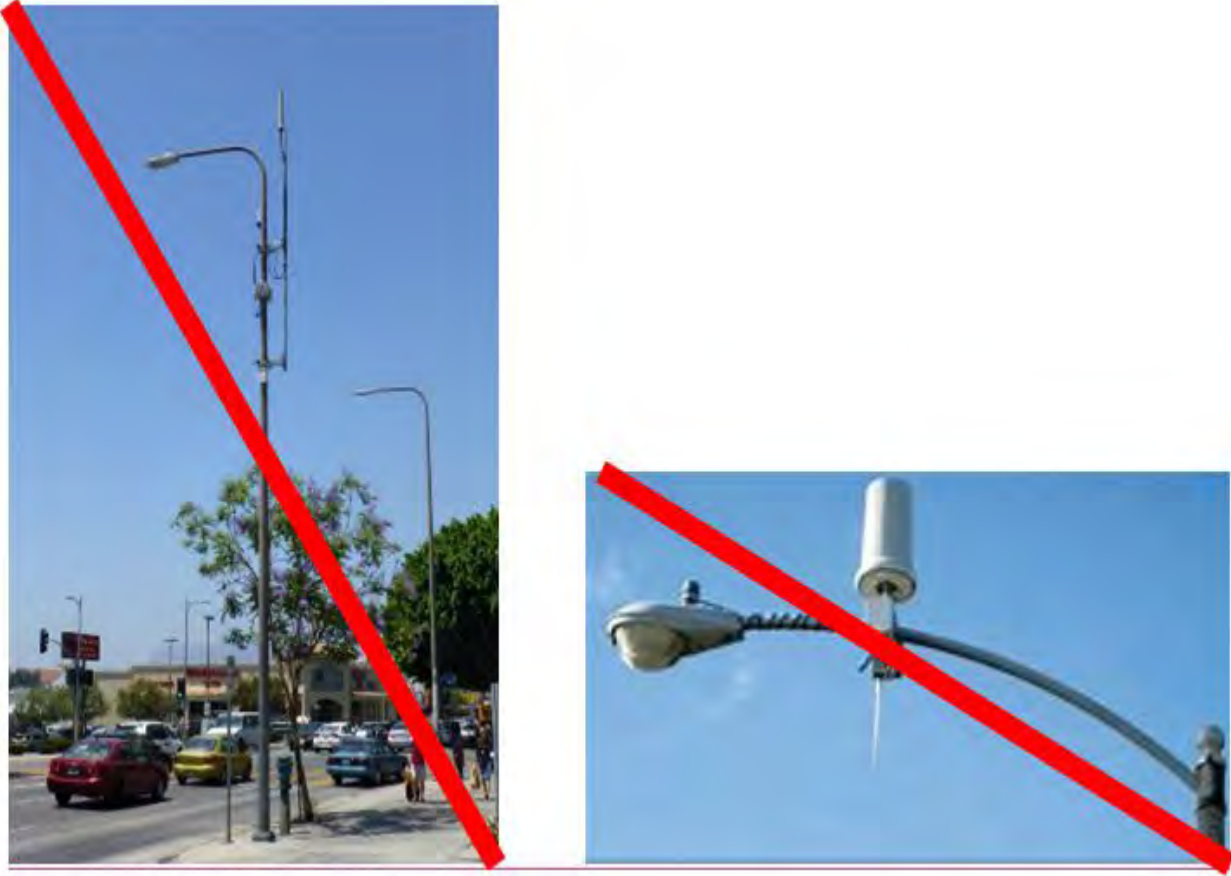
Figure 16.68.050(C)(4). Acceptable and unacceptable attachments
