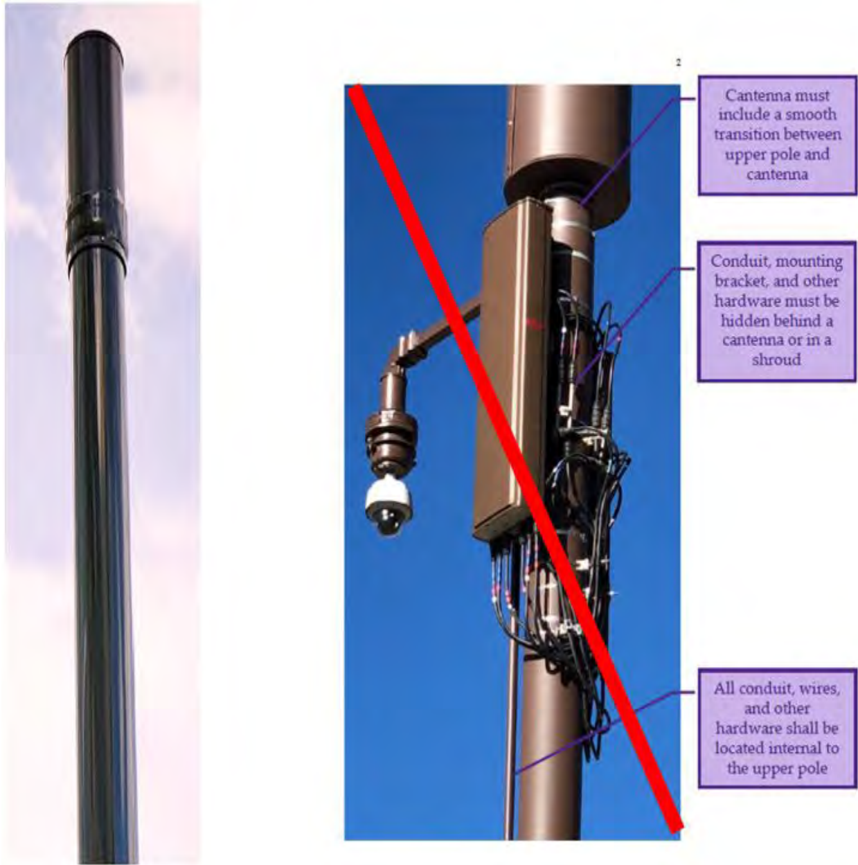
Figure 16.68.050(C)(5). Acceptable and unacceptable new poles
