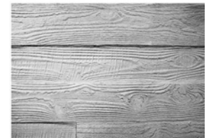
➤ Concrete wall texture
