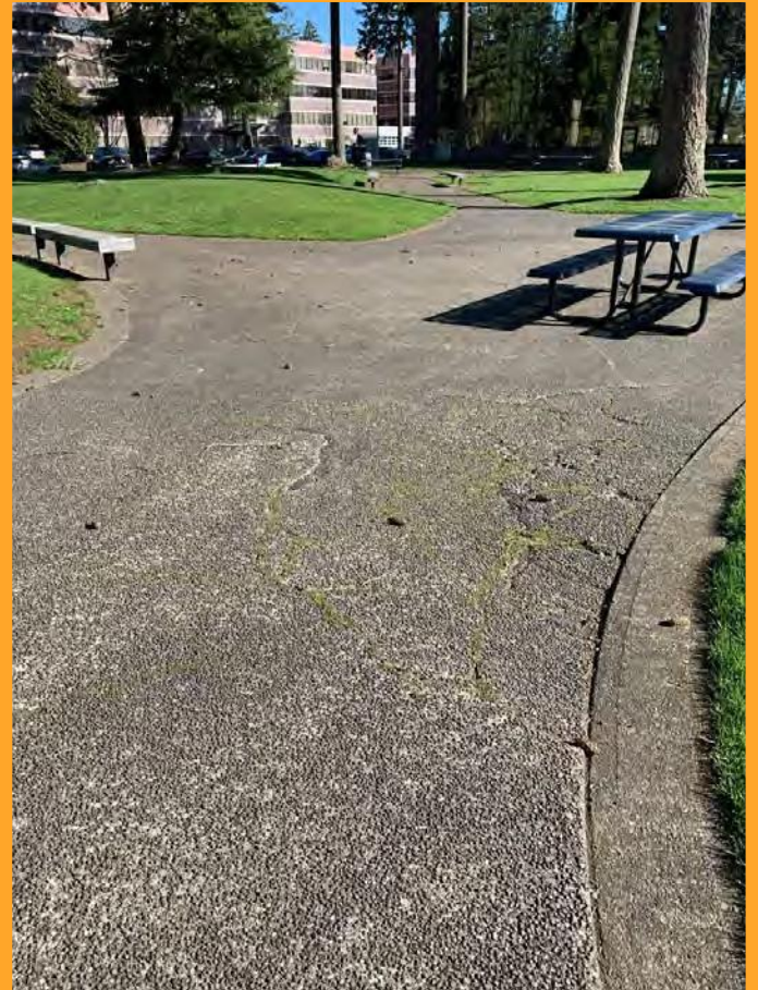
Large cracks
