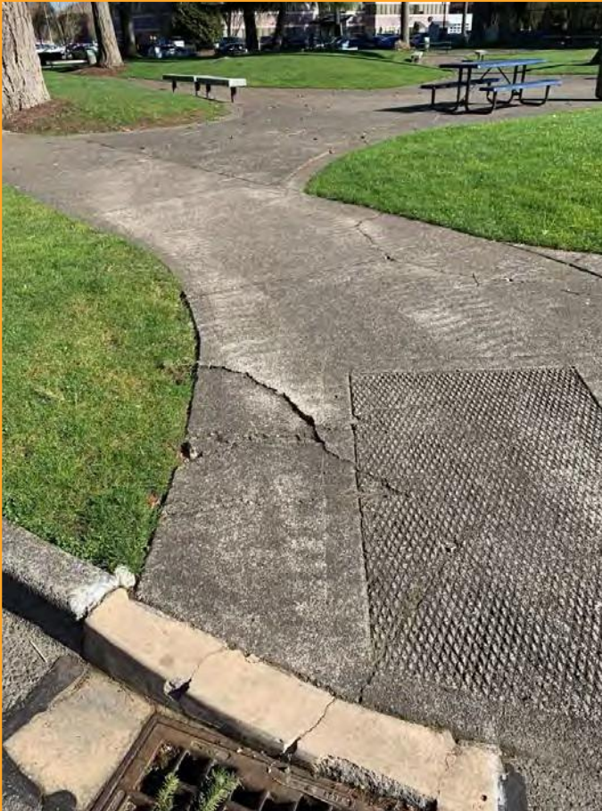
Large cracks
