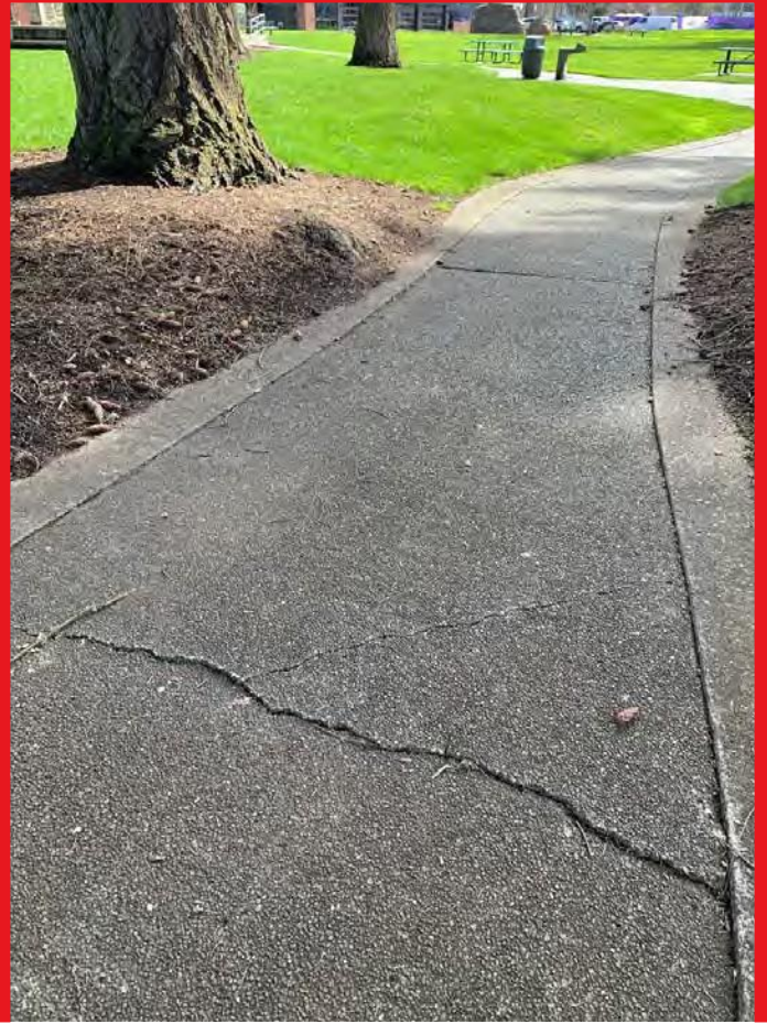
Large cracks
