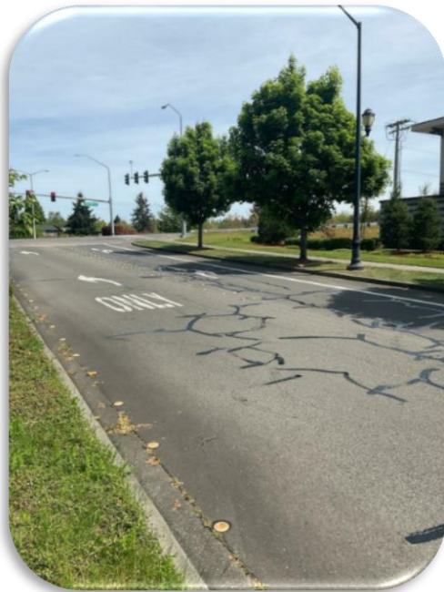
Balustrade Blvd SE
