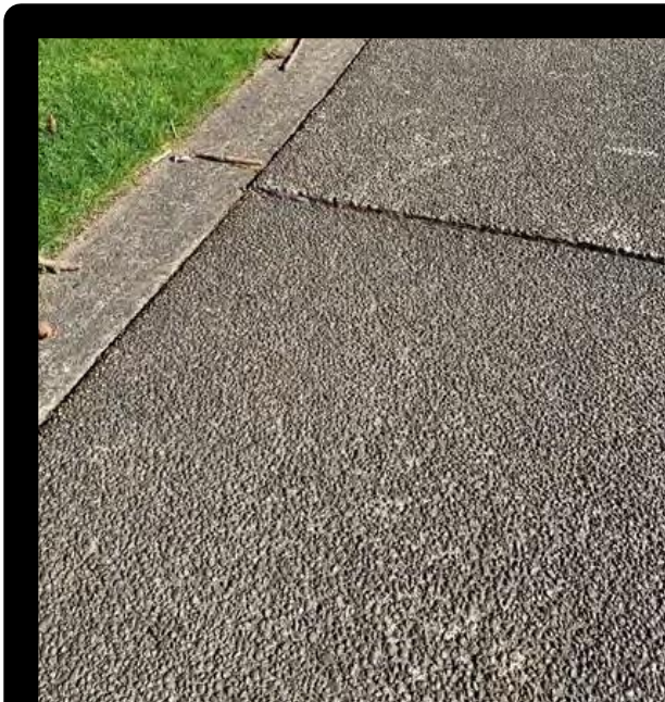
Photo of existing concrete design - aggregate with smooth border
