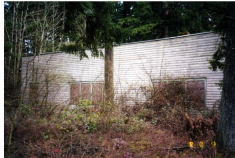
Exterior side, 2002.tif
