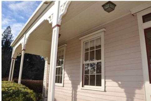
040 Front Single Pane Windows.jpg
