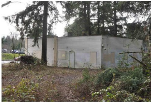
McKinney Building3 northeast corner showing side detail.jpg
