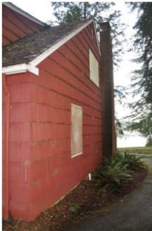
045 South side of house.jpg
