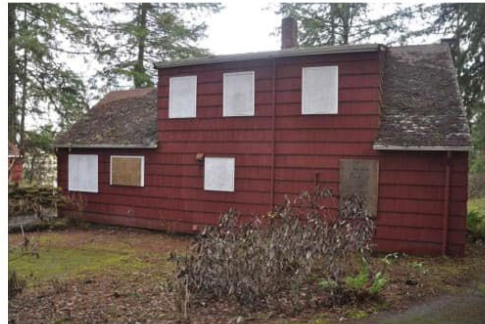
010 Back west side of house.jpg
