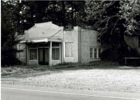
Lois McKinney House Apr 29 1987 (2).jpg
