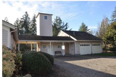
025 Back parking area, Add-on facing SW.jpg
