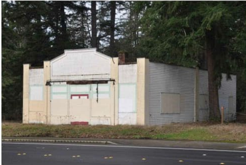
McKinney Building1 front facade, view facing north.jpg
