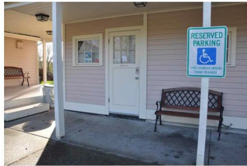
055 Tower Office Entrance facing SW.jpg
