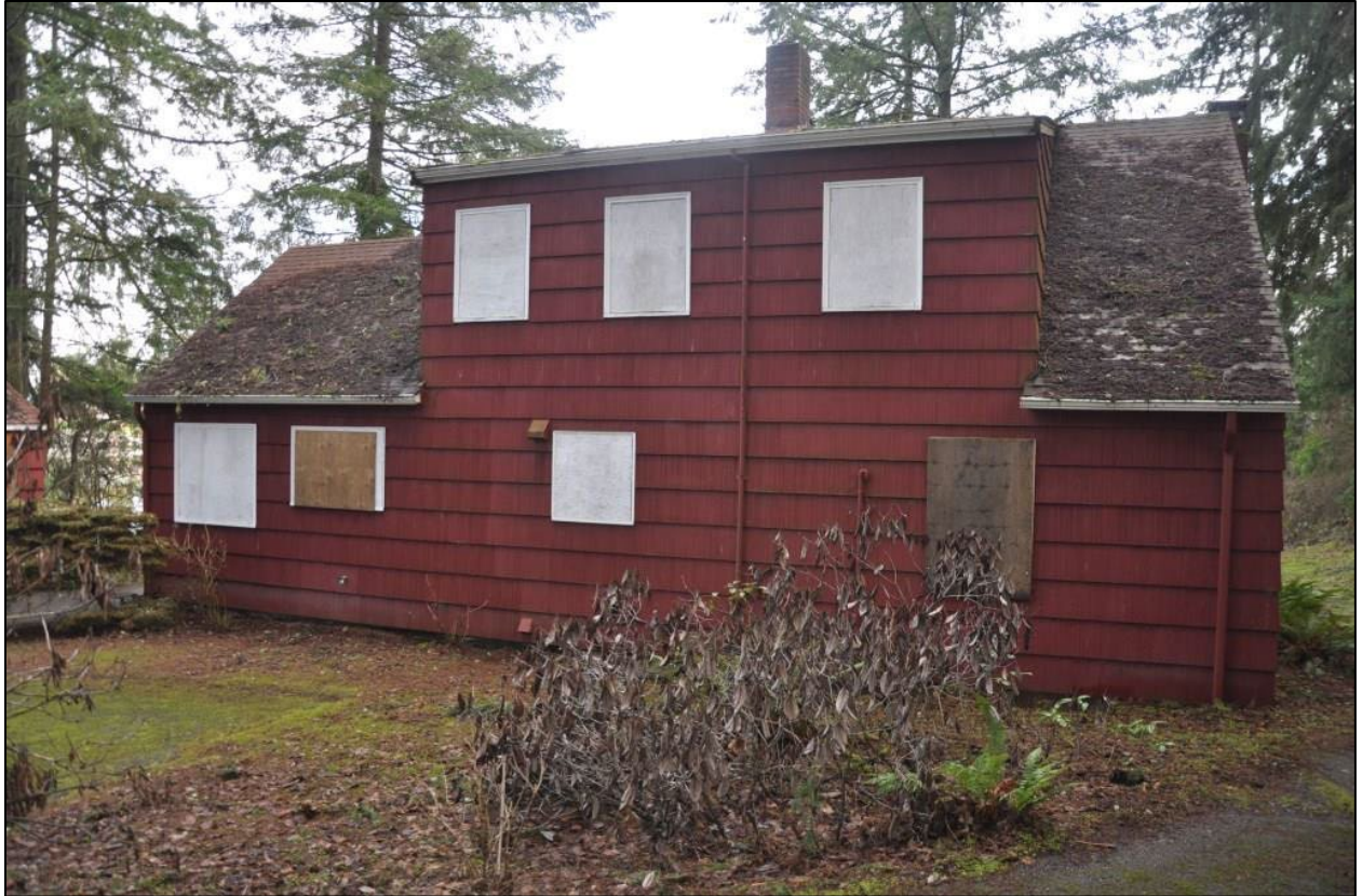
Photo 14. View of rear (west) façade, taken in 2025.
