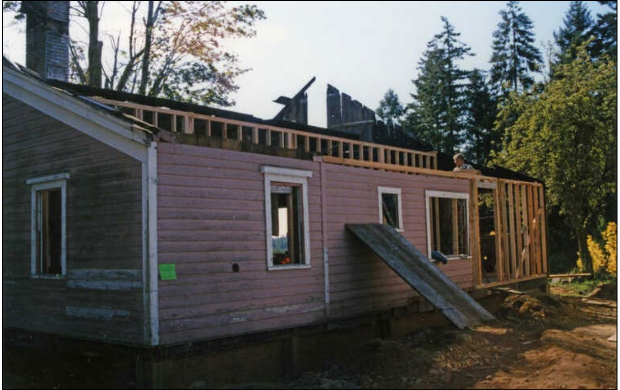
Photo 2. View of rear elevation, entire roof removed, taken in 1997.
