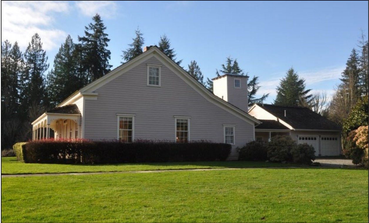
Photo 6. View of the east façade with water tower and detached garage. Taken February 2025.
