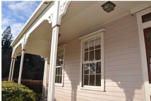
040 Front Single Pane Windows.jpg
