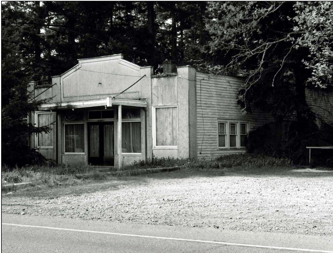
Photo 16. View of main (south) façade and east façade, taken in 1987.
