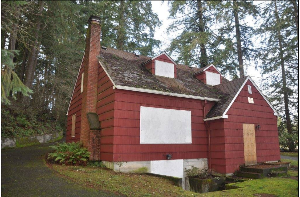
Photo 13. View of south façade, note full chimney, and main (east) façade. Taken in 2025.
