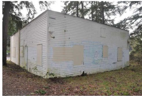
McKinney Building2 back of building, view facing southwest.jpg
