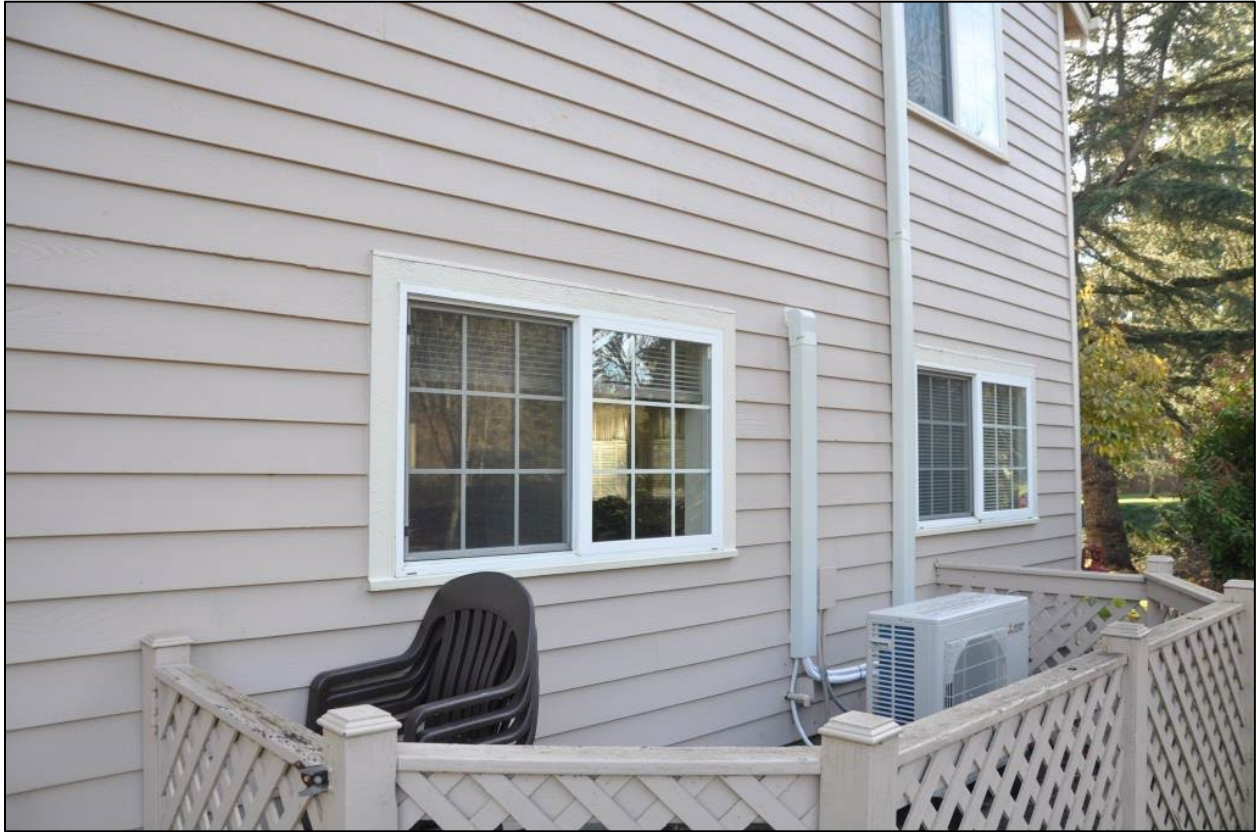
Photo 10. Modern vinyl windows on garage-apartment's rear (west) façade, taken in 2025.
