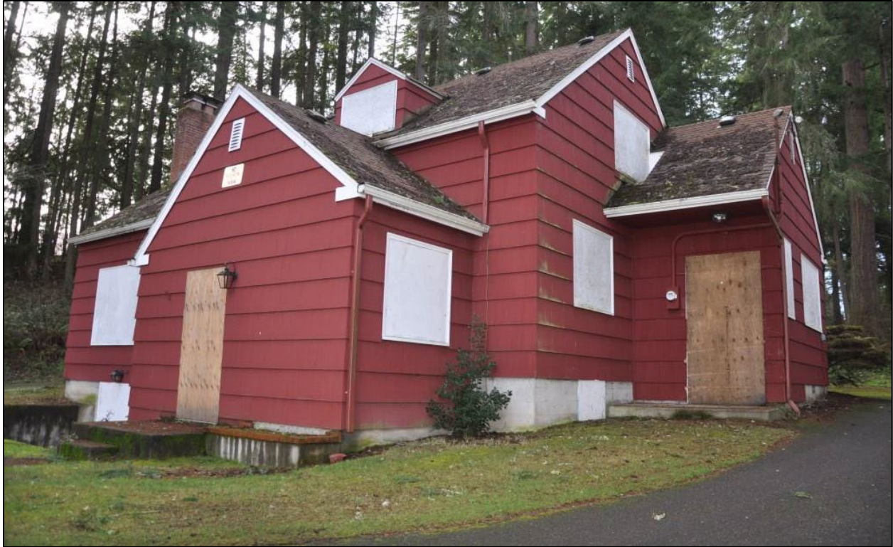
Photo 11. View of main façade (east) and north façade, taken in 2025.
