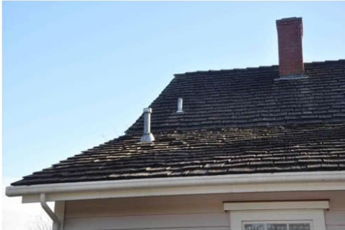
021 Roof of house.jpg
