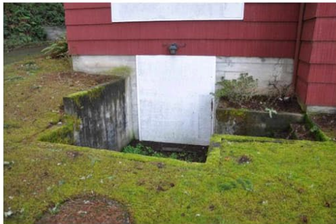
035 CloseUp of basement access.jpg
