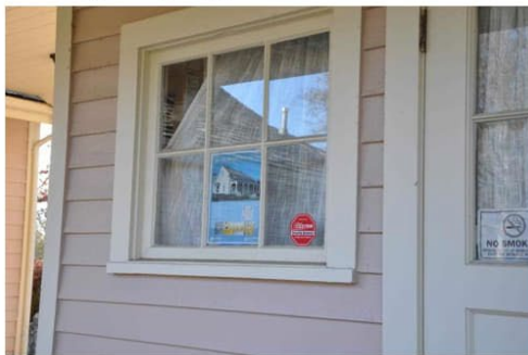
060 Tower Office Entrance CloseUp.jpg
