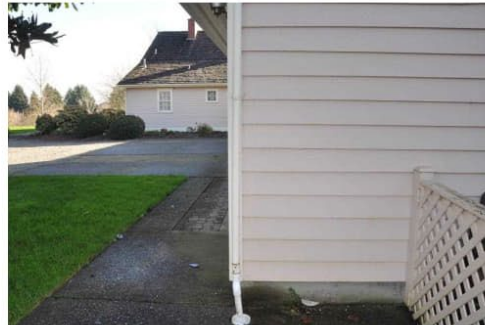
075 Garage facade SE for perspective.jpg
