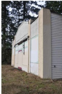
McKinney Building1.2 east corner of front facade closeup, view facing west.jpg
