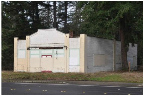
McKinney Building1 front facade, view facing north.jpg
