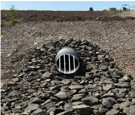
Construction of a Rock Splash Pad
