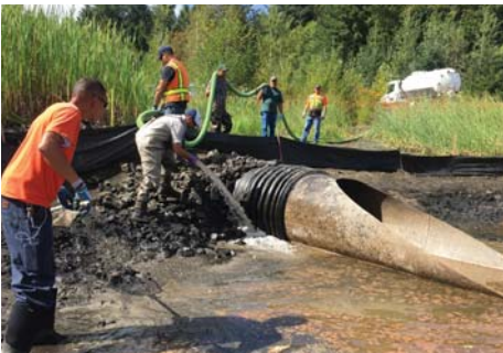
Maintenance Crews at College Regional Stormwater Facility
