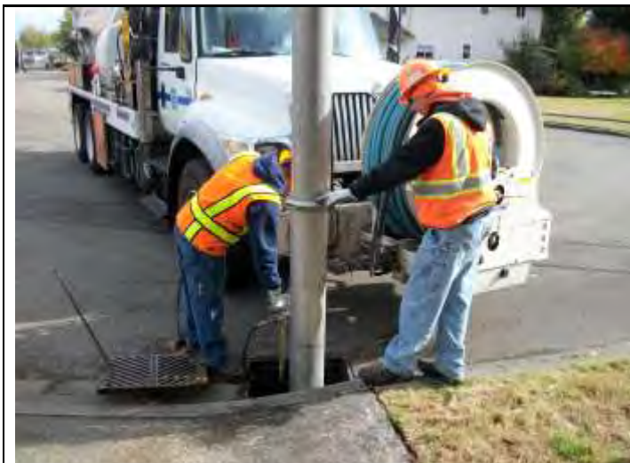
Catch basin cleaning
