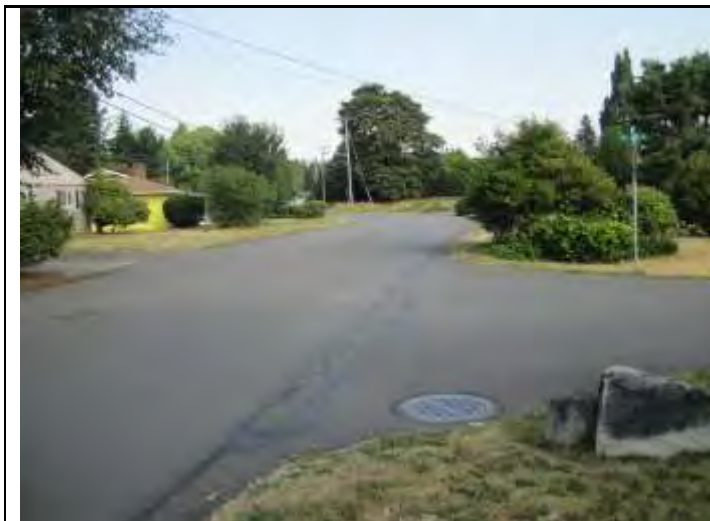
Neighborhood lacks stormwater drainage
