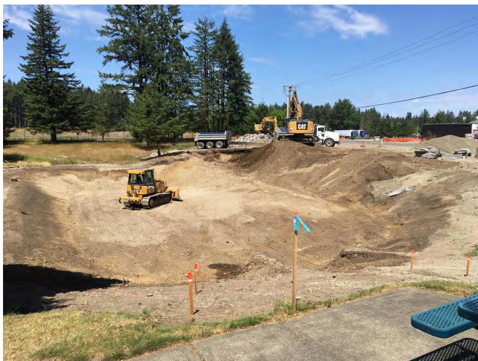
HOGUM BAY POND EXCAVATION
