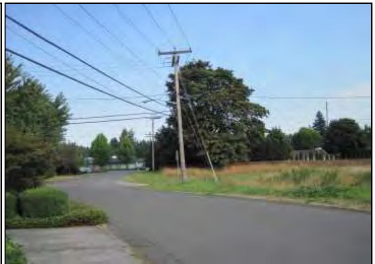
Neighborhood lacks stormwater drainage
