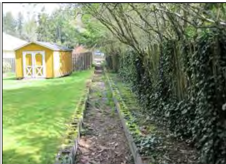
Existing above-ground overflow from facility.
