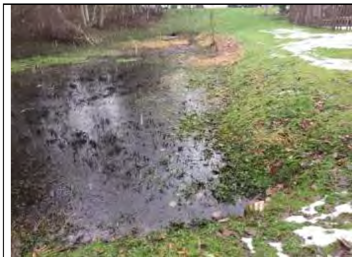
Existing stormwater pond, looking north
