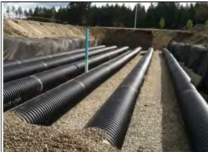
Infiltration gallery construction
