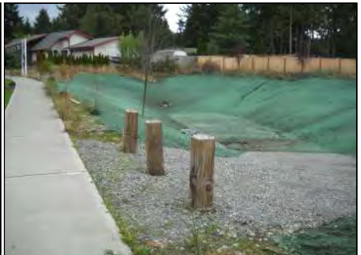
Facility under construction
