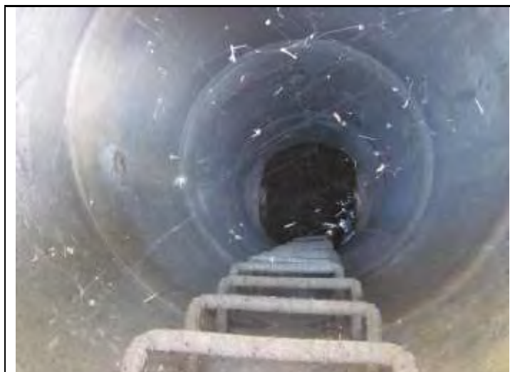
Existing structure access
