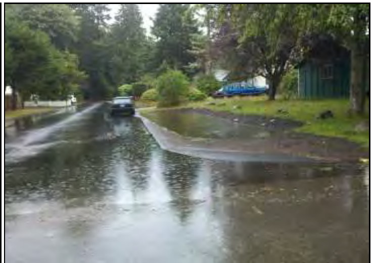
Road without drainage system
