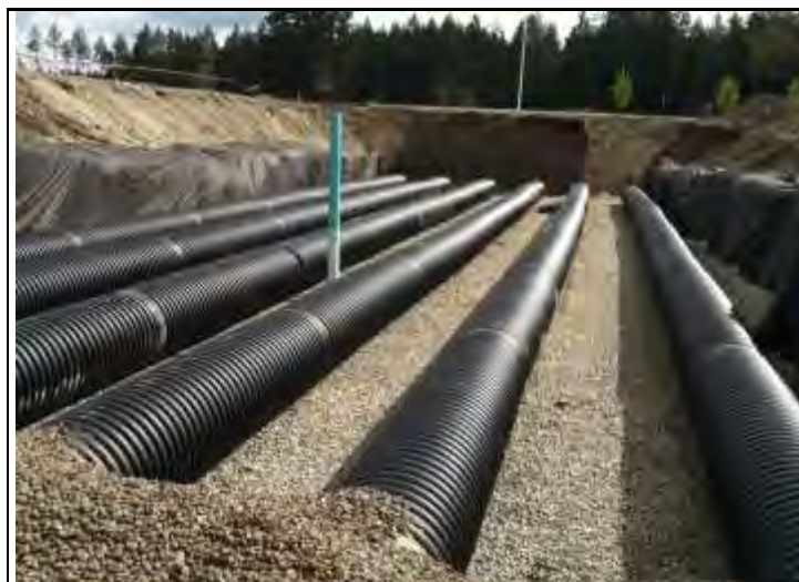
Infiltration gallery construction
