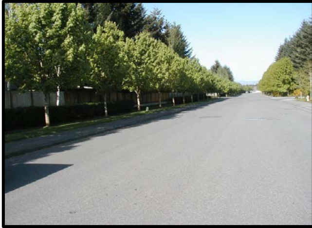
Photo D. View of privately maintained street trees in SE Lacey. A case where trees are well-maintained.
